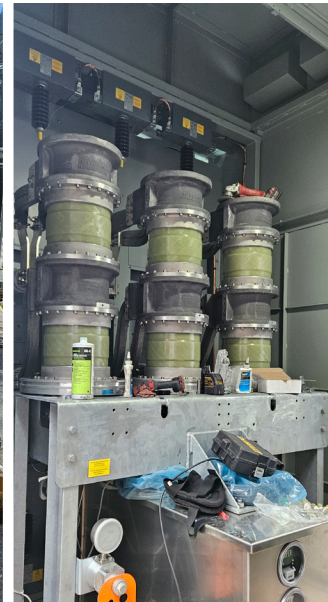
Left to Right: Unwrapping second new breaker prior to installation.
