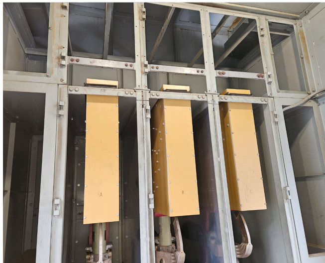
One of the two existing breakers prior to removal.
