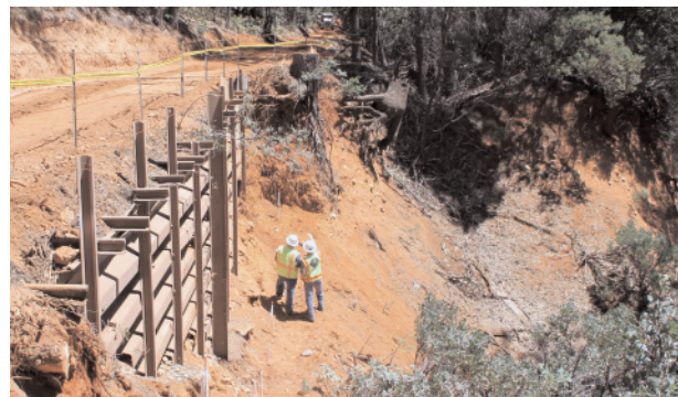
The Gold Run project includes a 96-foot-long retaining wall, seen here in construction.
