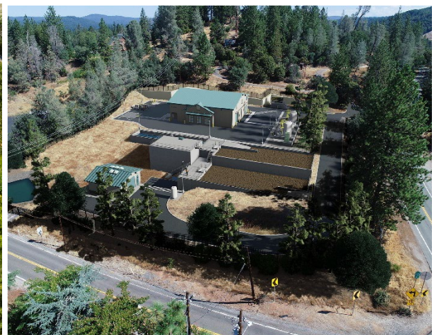
This rendering shows the future Colfax Water Treatment Plant, designed to meet the growing needs of Colfax and nearby communities with modern, efficient water treatment.
