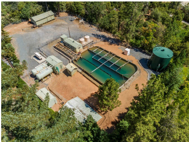
Built in 1958, the current Colfax Water Treatment Plant has served the community for decades. A new facility will take its place to provide more reliable water for the future.
