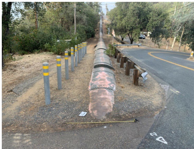
PG&E's Penstock in the Duncan Hill community.
